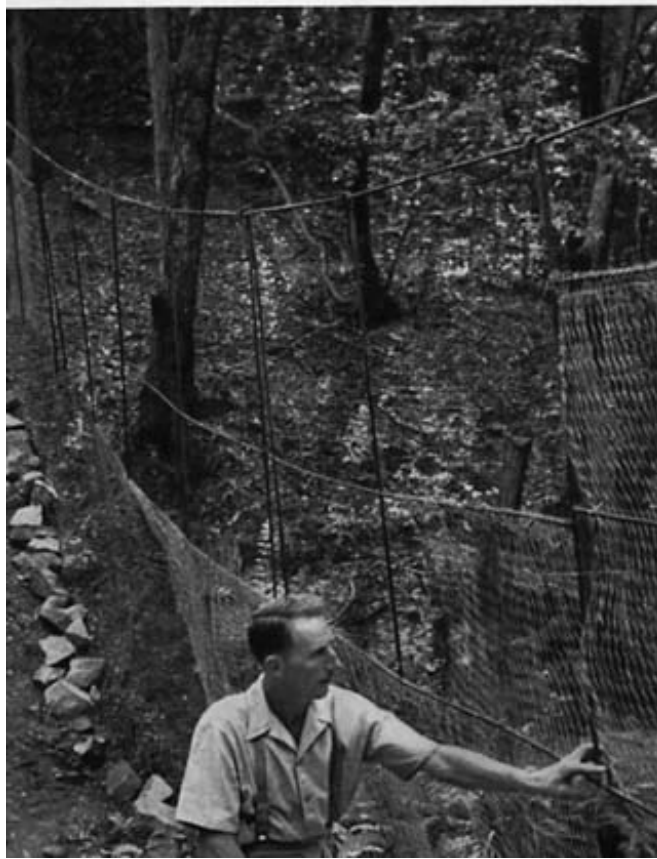
Plate 9: Jack Matters and a rabbitproof flood-gate he built. Held down with rocks, flood-gate swings out with the floods. Jack is in charge of the two properties.
