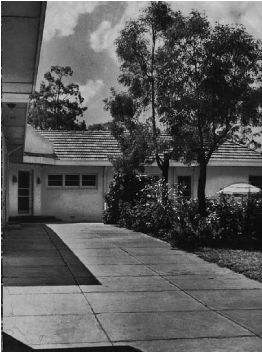
Plate 15: "Nevallan" homestead is of cavity wall construction, cement tiles and bricks made on the property. Insulated against heat and cold, protected from flies and mosquitoes, it has the conveniences and modern comforts so necessary for country as well as city living.
